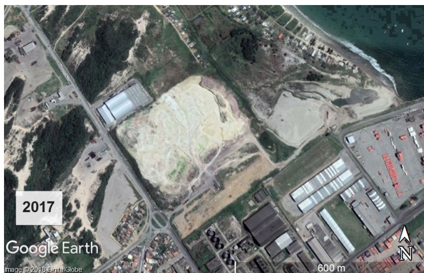
Figure 13: Phosphogypsum stack 2 at Imbituba in 10/23/2017
