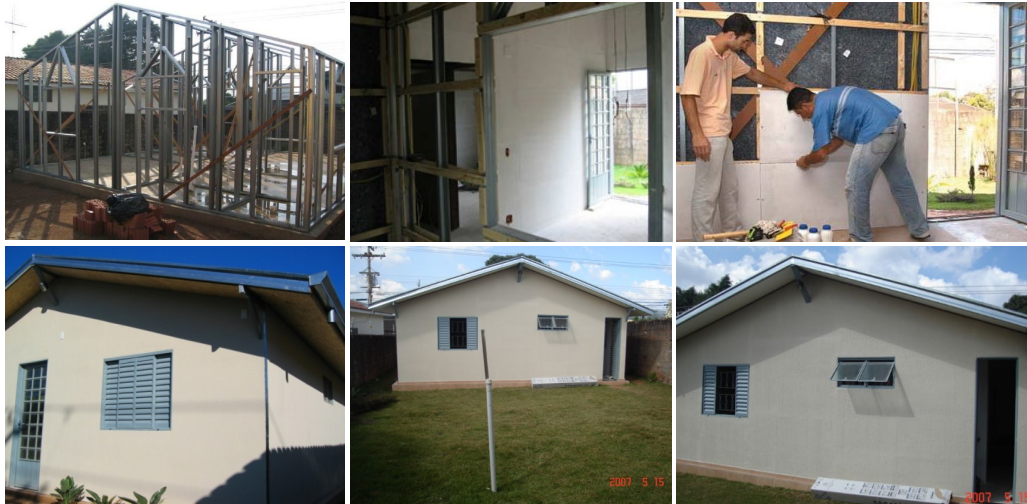
Figure 18: Experimental house built with phosphogypsum plates
