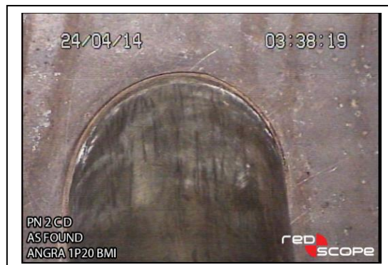
Figure 8: Angra 1 Reactor Vessel Bottom penetration.
