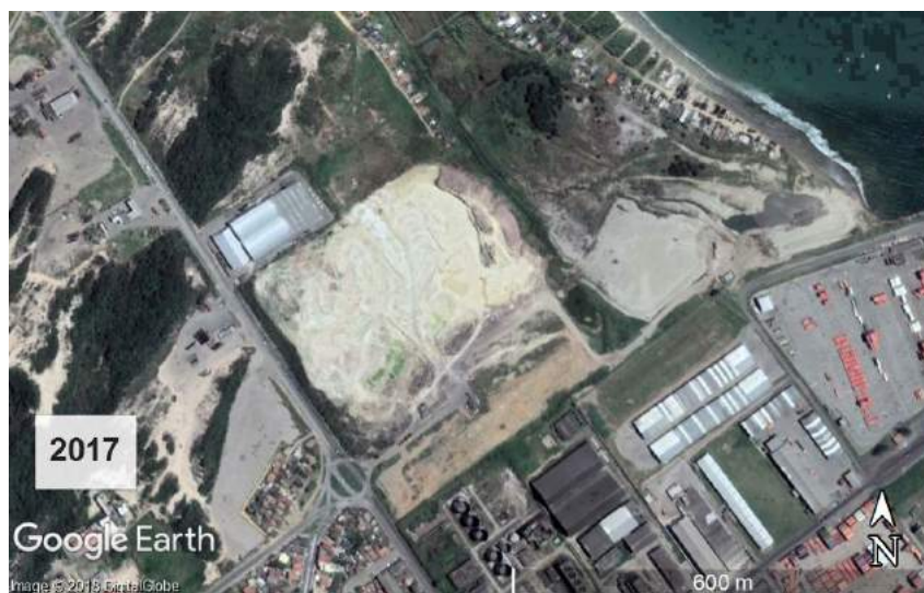
Figure 13: Phosphogypsum stack 2 at Imbituba in 10/23/2017
