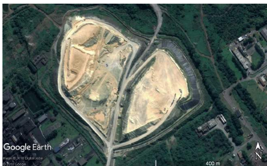
Figure 6: Phosphogypsum stack at Cubatão phosphate fertilizer complex (owed by CMOC) in 06/16/2017
