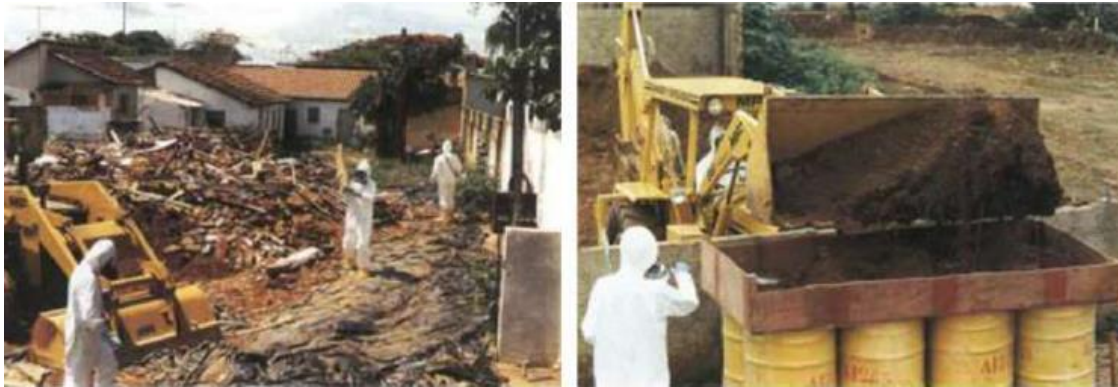
Figures 2 and 3: Decontamination work by CNEN teams - Goiânia, 1987.
