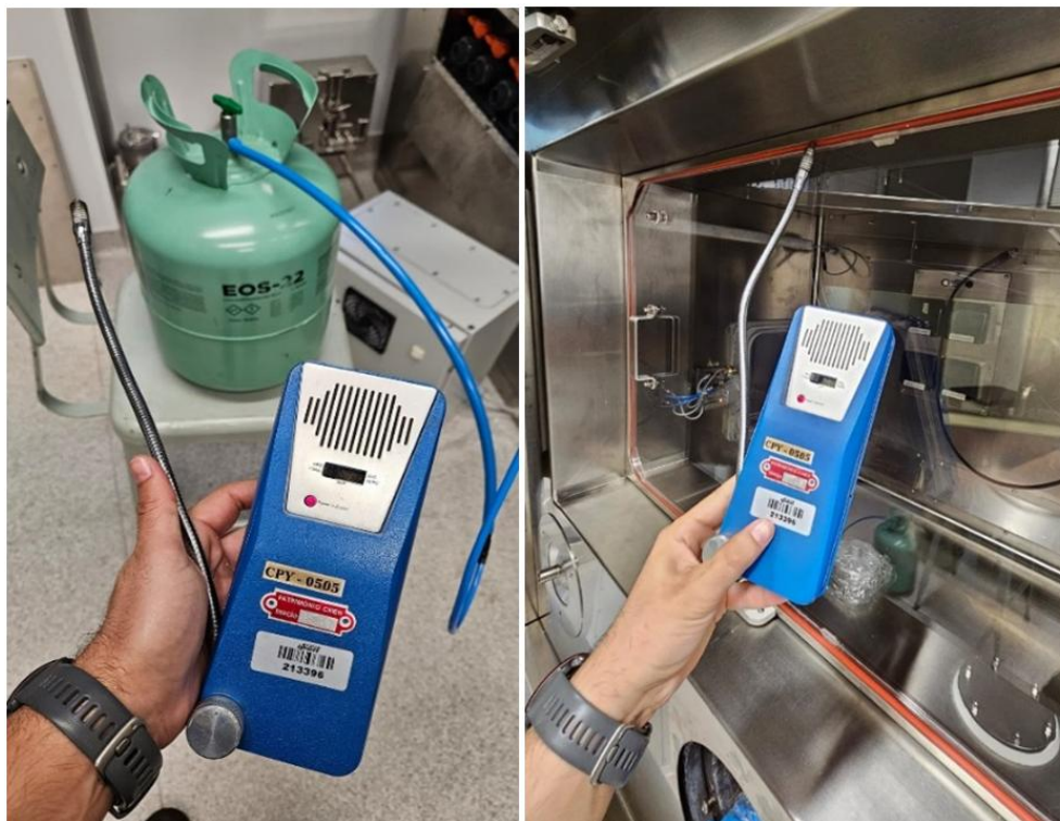
Figure 4: Leak detection with refrigerant R22.
