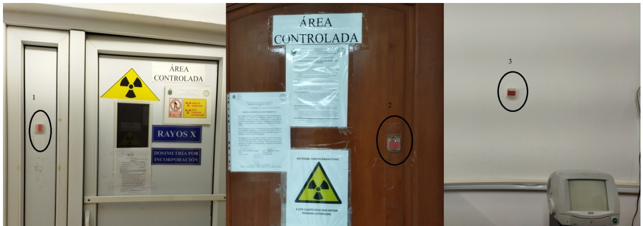
Figure 3. Example of three measuring points with the TLD arrangement. Photo in the left indicates the dosimeter placed at the entrance door of the area of LCM where the mobile X ray is located, photo in the center shows the dosimeter place at the entrance door of the source storage room and photo in the right side depicts the dosimeter place at the wall between the bunker and the control room in LCD.
