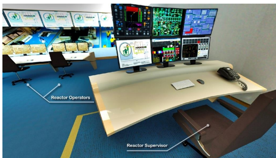
Figure 2: The Main Control Room
